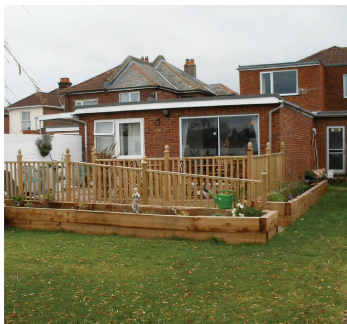
Avondale before the renovations began
